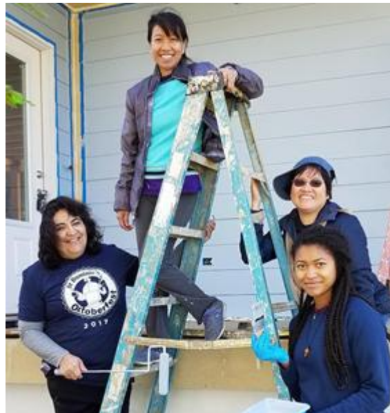
Working on a house for the St. Bernard Project.
